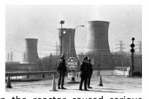
in 1979. Overheating in the reactor caused serious damage to fuel rods and created a pressure rise in the system. Valves were opened to lower this pressure, but they failed to close again and released radioactive material into the environment. Want to know more about the accident? Watch this video: Moments in NRC History: Three Mile Island - March 28, 1979
